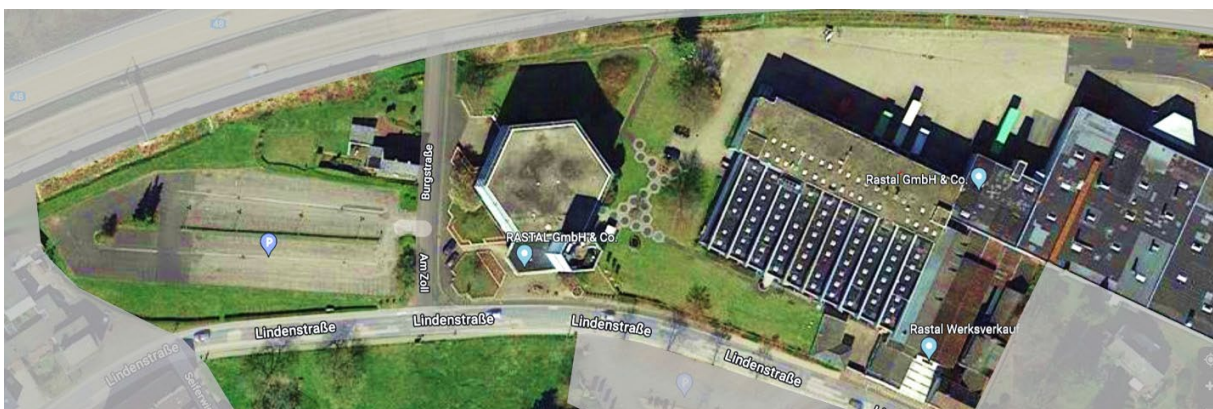
RASTAL Factory Premises - Höhr-Grenzhausen, Germany
